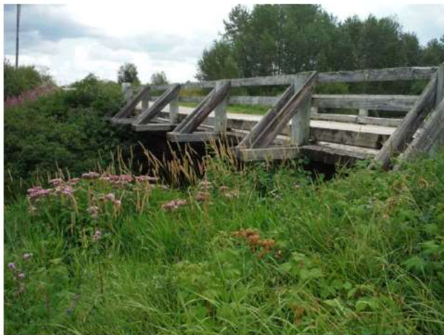
6- View of north side of bridge
