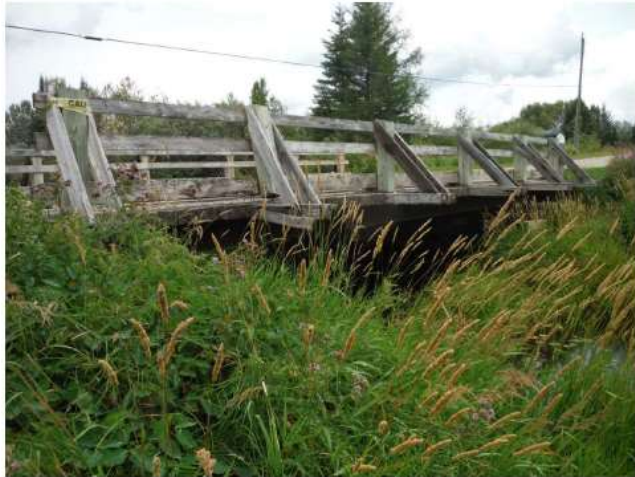
5- View of south side of bridge
